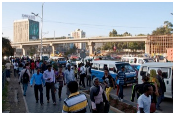
Fig. 18: Light Rail under construction, pedestrian traffic in morning rush hour, C. Pardo 2014
