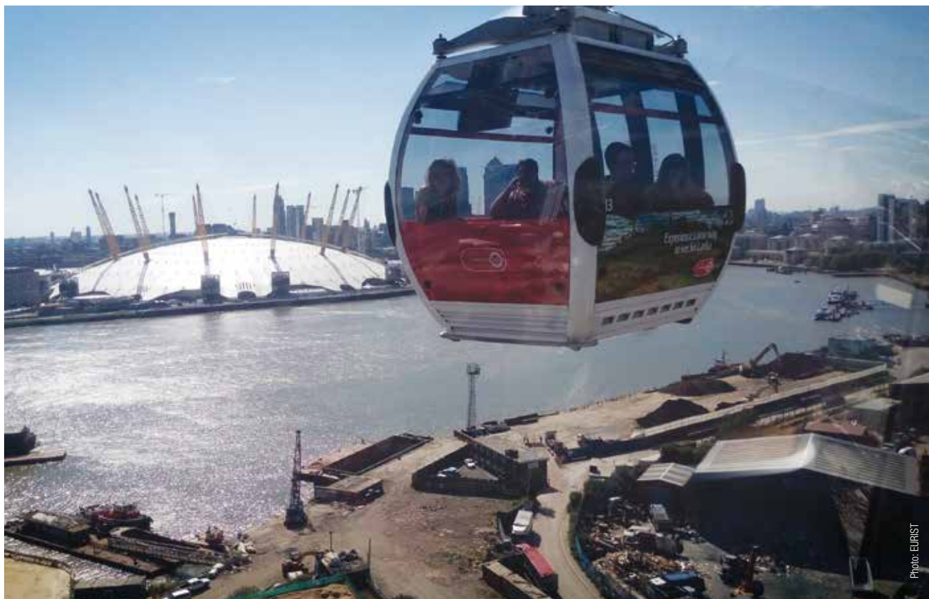
The Emirates Air Line bridges the Thames, running 90 metres above the ground, connecting north and south London
